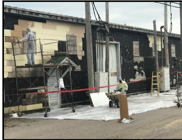
Asbestos abatement on the exterior siding of a warehouse. Located on the MağWakçaçk "Sacred Earth" / Former Badger property.
