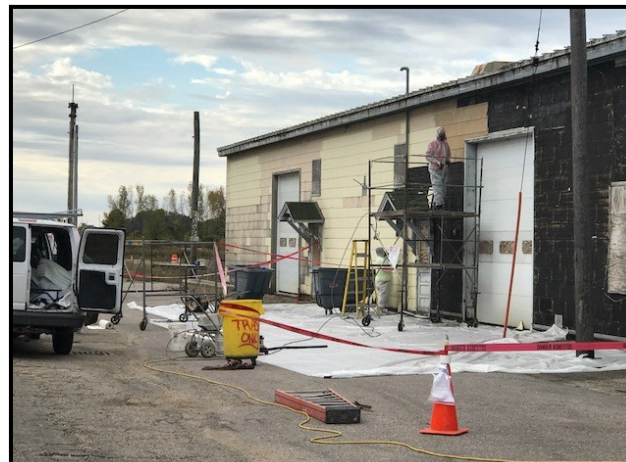
Asbestos abatement on the exterior siding of a warehouse. Located on the MağWakçaçk "Sacred Earth" / Former Badger property.
